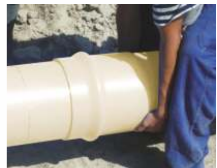
Align the pipe and place the spigot end inside the socket or bell.
