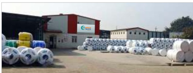
Manufacturing Plant - Sikandrabad (U.P.)
