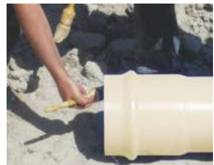
Apply lubricant on the chamfer of the spigot end and in the rubber ring joint.
