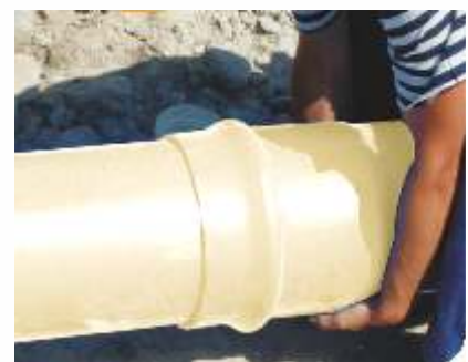
Firmly push the free end into the other pipe. Introduce until the end marked is no longer seen.
